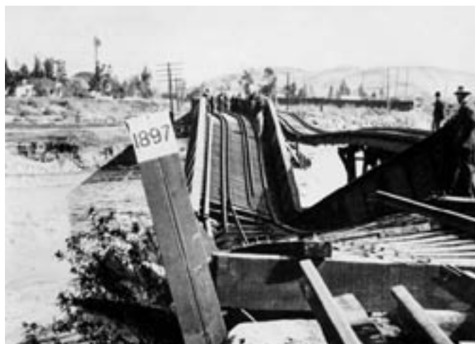
Figure H-7. Railroad Bridge Washout, 1914 (Los Angeles Public Library)
