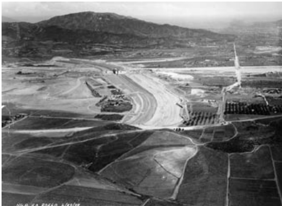
Figure H-8. Construction of Hansen Dam, 1939. (San Fernando Valley Historical Society)
