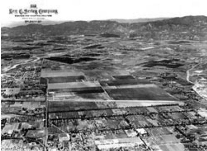
Figure H-11. Panorama Ranch 1946, with Tujunga Wash on right, Pacoima Wash on left. (Los Angeles Public Library)
